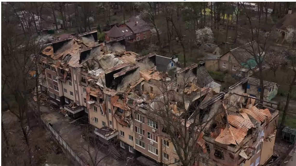
Damage to apartment blocks in Irpin video
